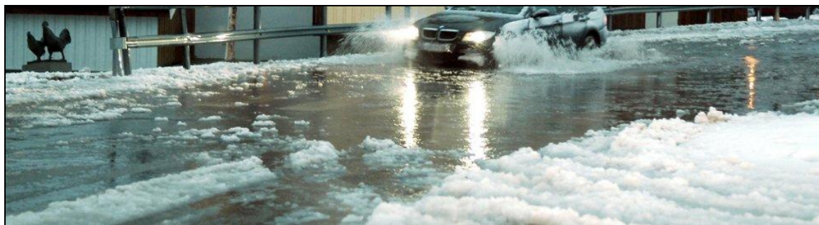
Figure 7: Typical late winter situation in Trondheim, when ice and snow are blocking the ducts and the water accumulates in the roads.
