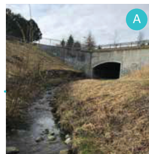
Tunnel under Bromstadvegen
