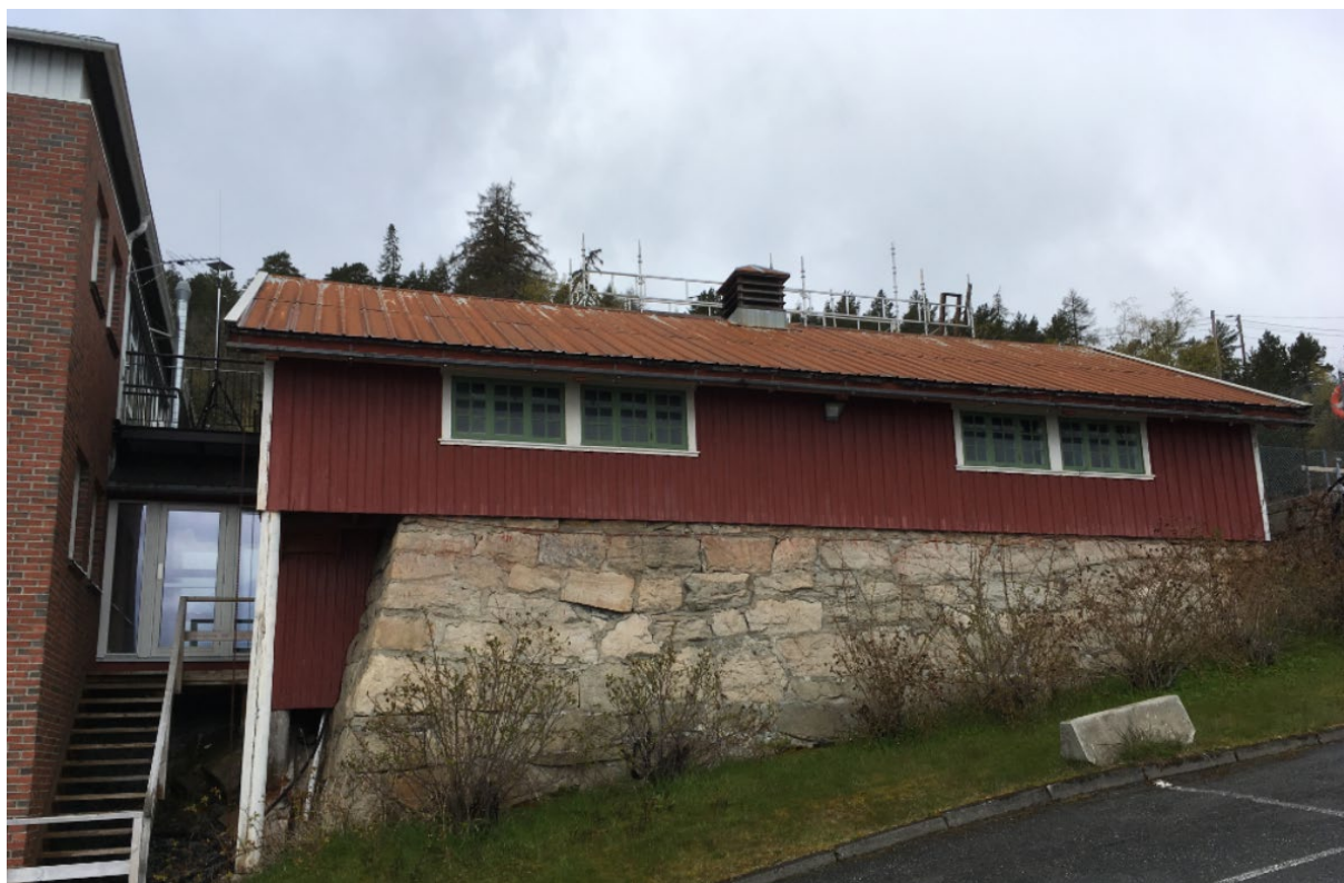
Figur 12; Klekkeriet (Foto: Gottlieb Paludan Architects 2020)
