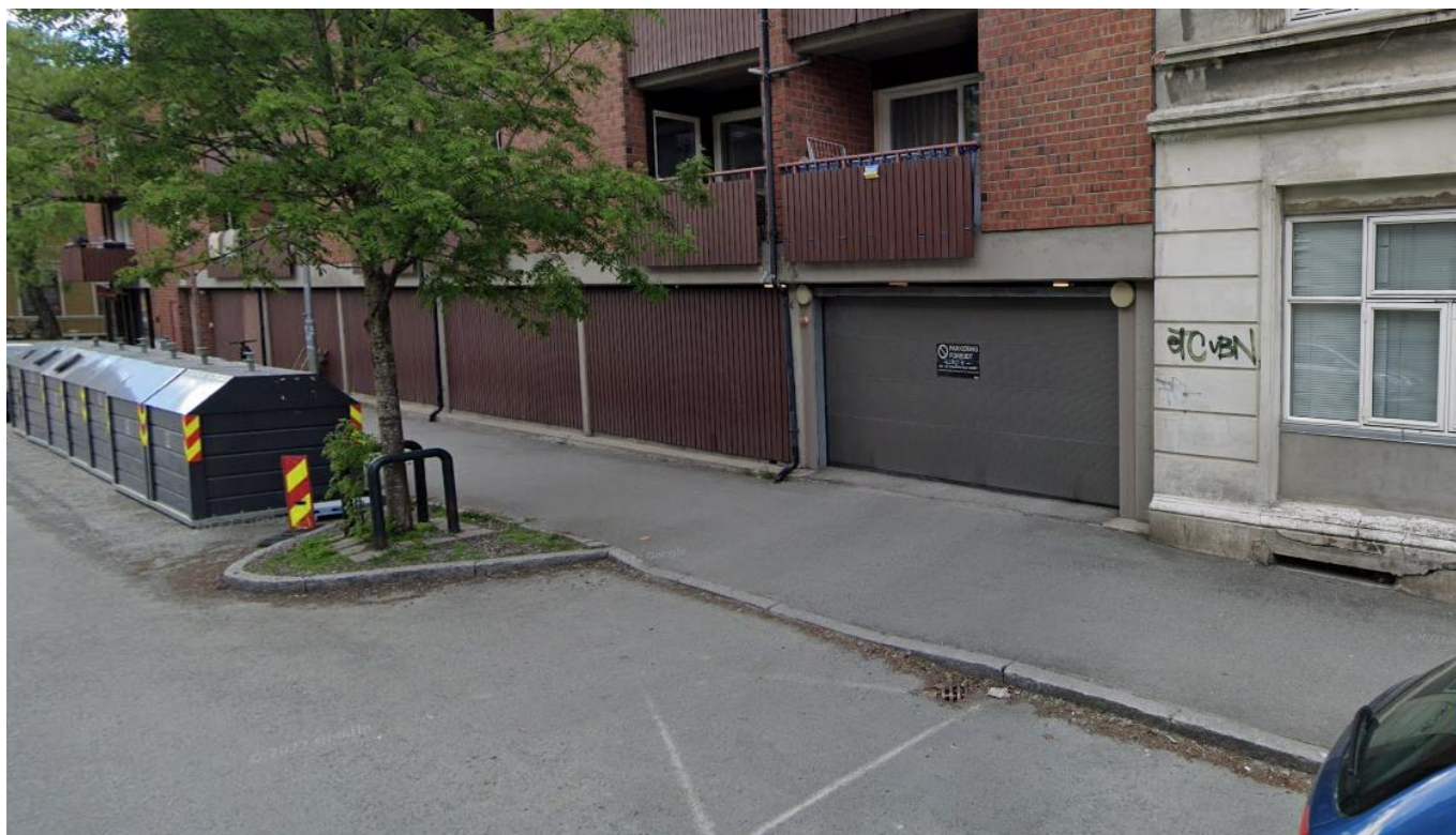
Figur 5 - Garasje i Abelsborg gate, Google Street View
