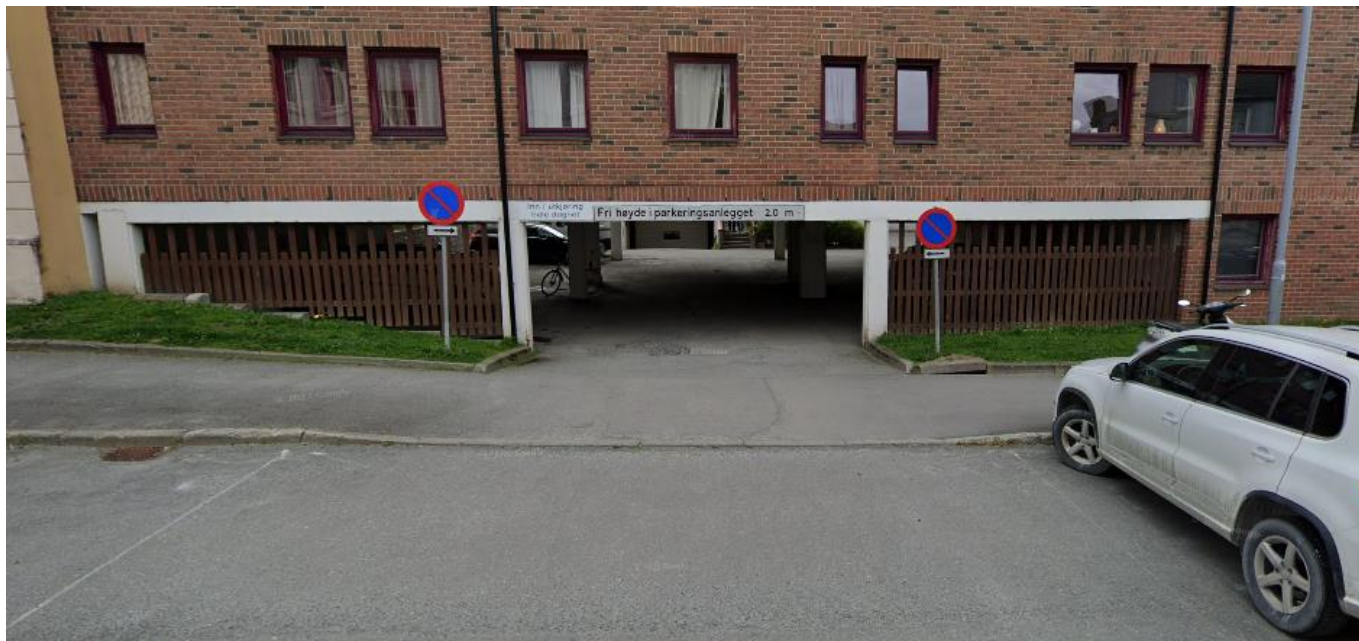
Figur 6 - Ila garasje, Google Street View
